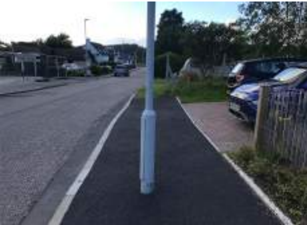
Lamp post in middle of pavement
