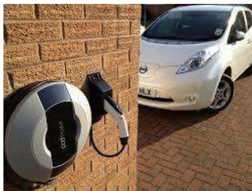
Figure 4: Wall-mounted universal EV charger 16
