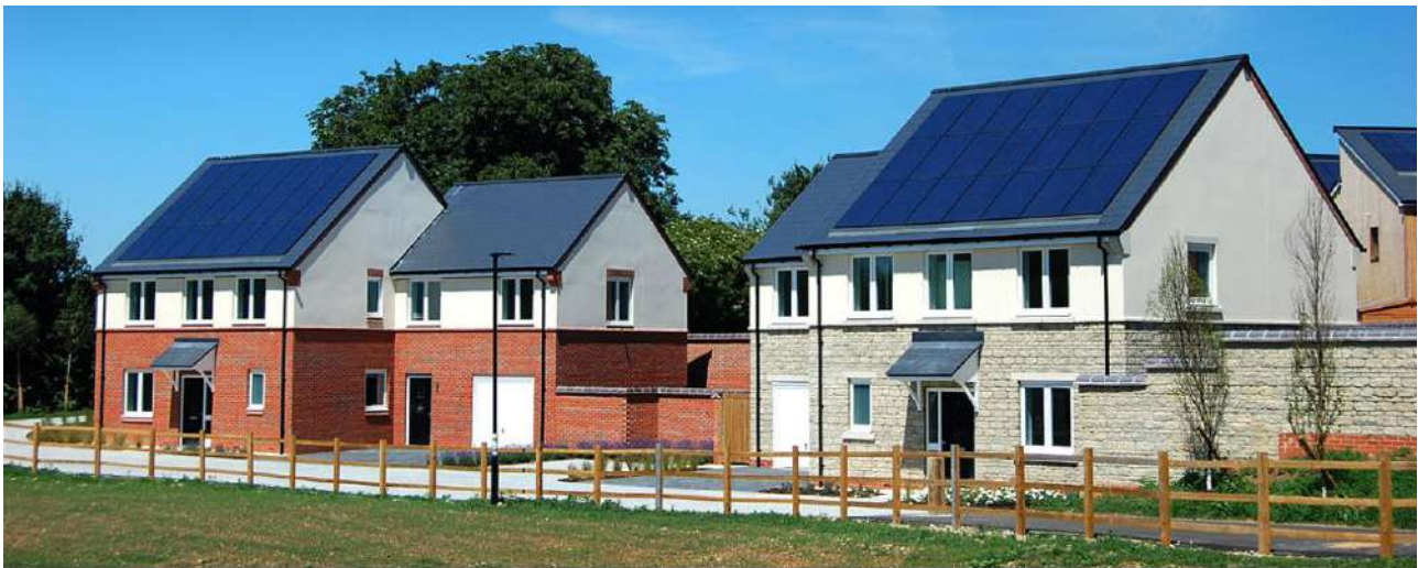
Figure 1: Roof-integrated Viridian solar PV arrays 11
